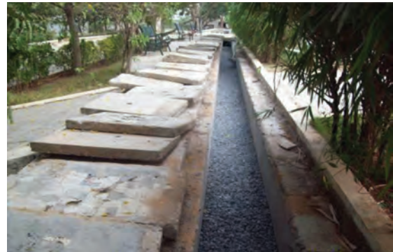
Rainwater recharge trench
