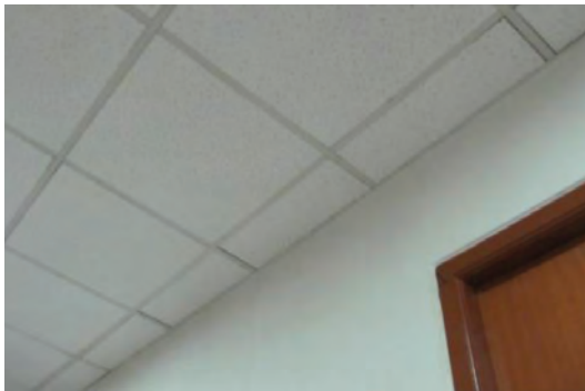
Reuse of excess ceiling tiles for edges
