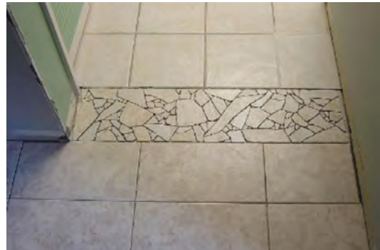
Reuse of broken floor tiles for edges / transitions / to provide relief
