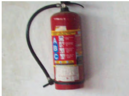
Fire extinguisher with ABC dry chemical
